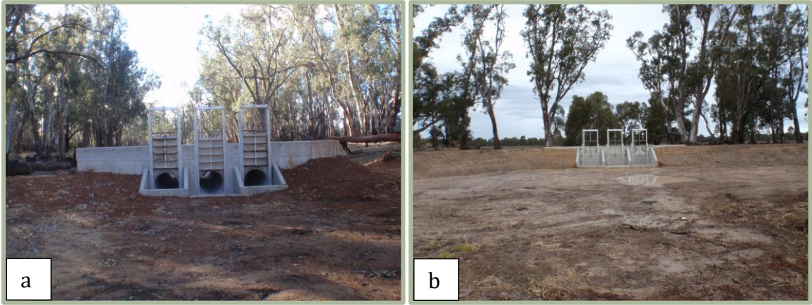
Figure 8: Warrigal regulator upgrade (a) and Yambuna regulator upgrade (b) in 2010.
