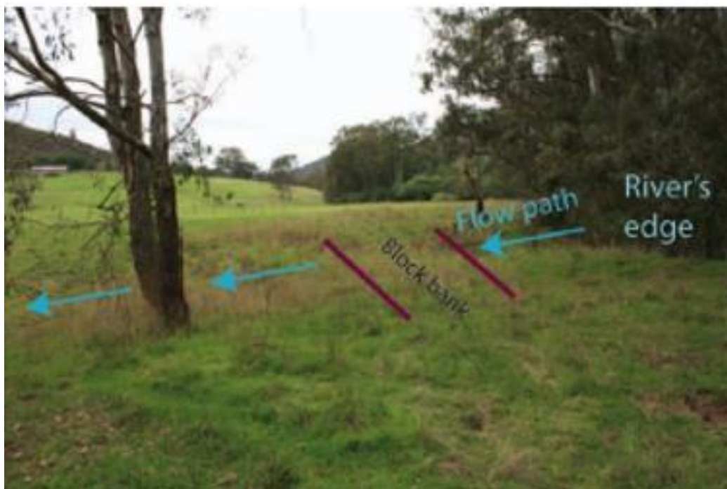
Figure 6: Block bank reducing inflows to a floodrunner immediately upstream of Horseshoe Lagoon (Photo taken by G. Vietz in Cottingham et al., 2014)
