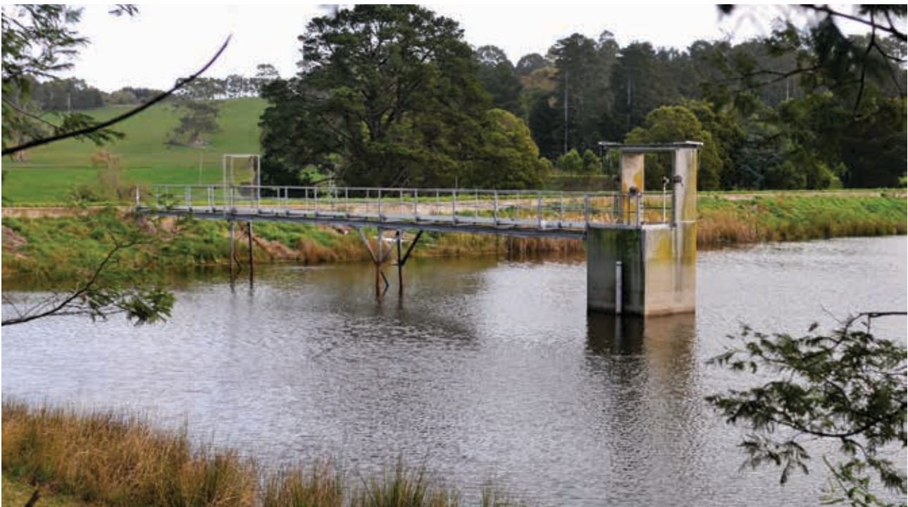
Korumburra water treatment
