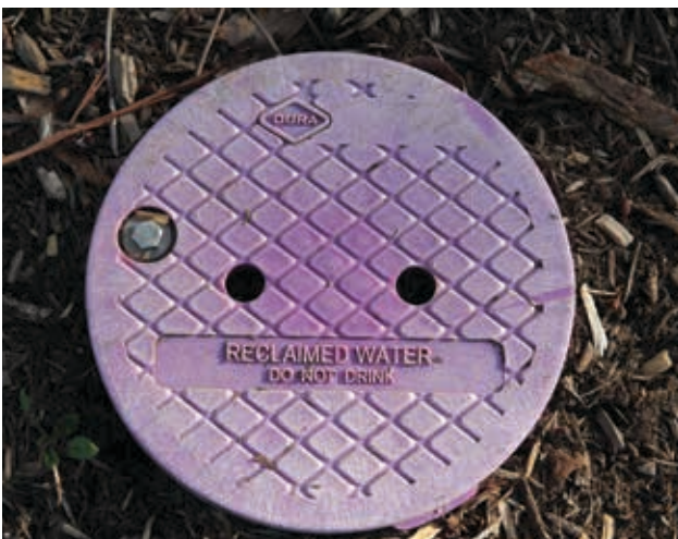
Coliban water pipe
