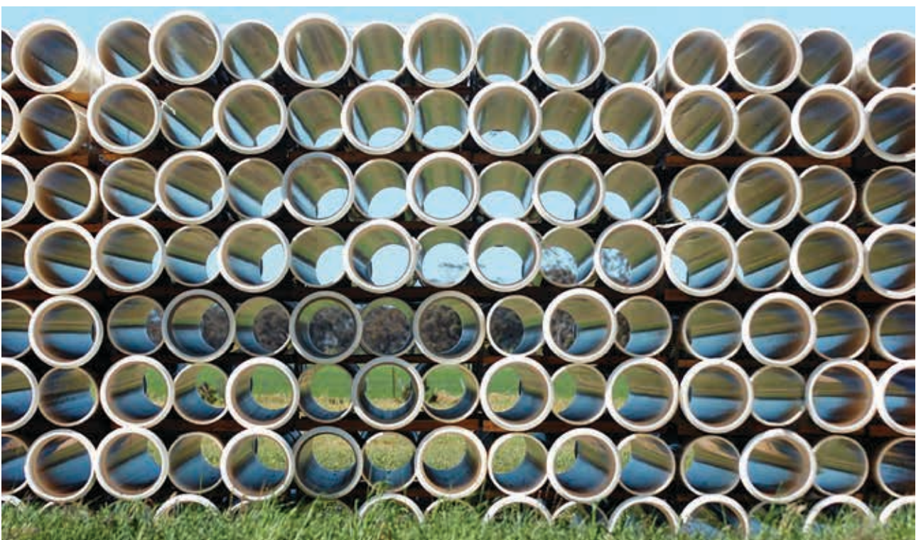
Pipe stack pile, WMPP Construction
