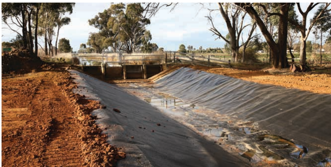
Channel Lining, Central Goulburn channel
