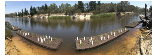
Floating wetlands along the perimeter of the Weir Pool have been installed by Wimmera CMA to help prevent bank erosion and ensure the integrity of the site in the longer term. Courtesy Wimmera Catchment Management Authority.
