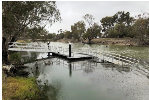
TOP: Dimboola Rowing Club pontoon. BELOW: Canoe launching facility at Horsham Weir Pool. Courtesy Wimmera Catchment Management Authority.
