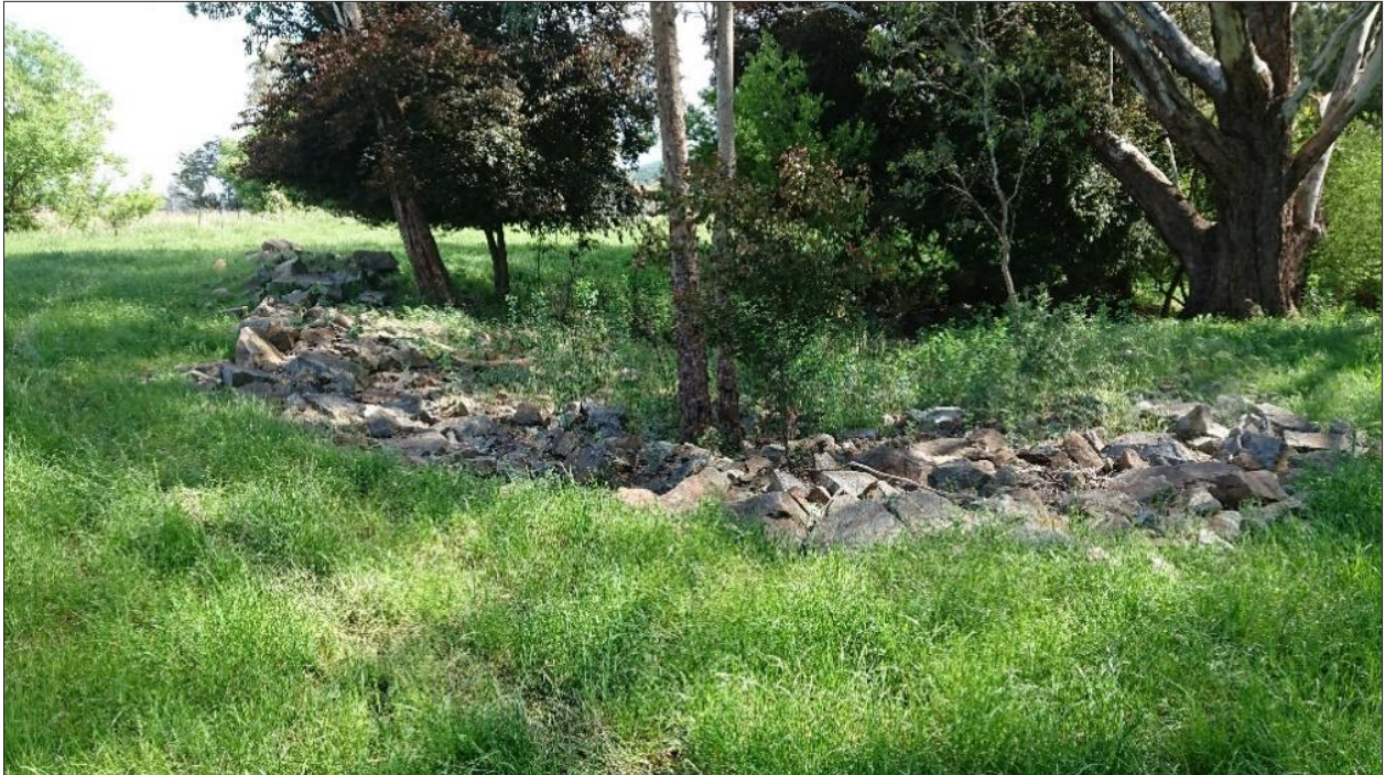
Figure 32. Rock work installed at the upstream end of a developing floodplain channel that conveys flow from the Owens River (parent channel) to Happy Valley Creek (daughter channel).
