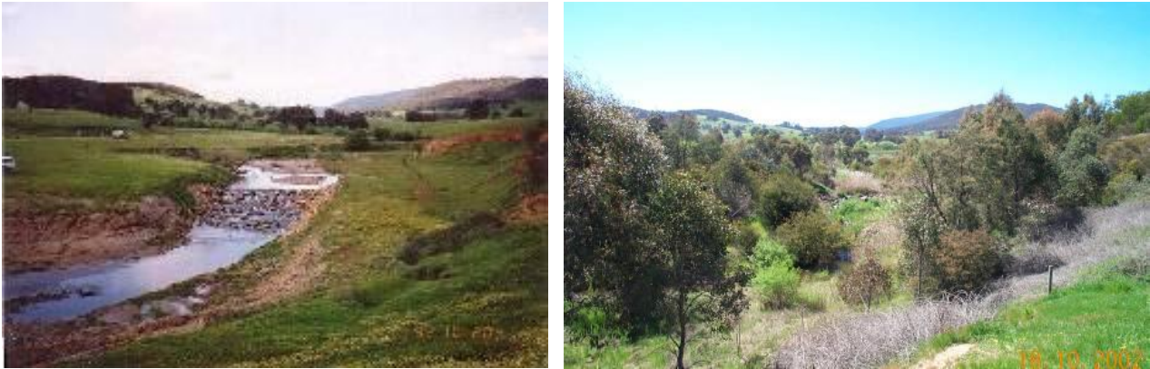
Figure 70. Barwidgee Creek, north east Victoria, six months (left) and 10 years (right) after rock chute construction and revegetation (Images courtesy of T. McCormack, North East CMA).
