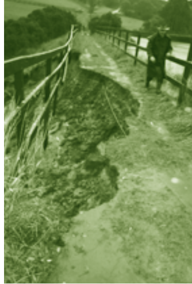
PHOTO COURTESY OF MELBOURNE WATER
