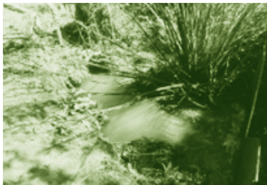
Leakage – measurable flow of water
